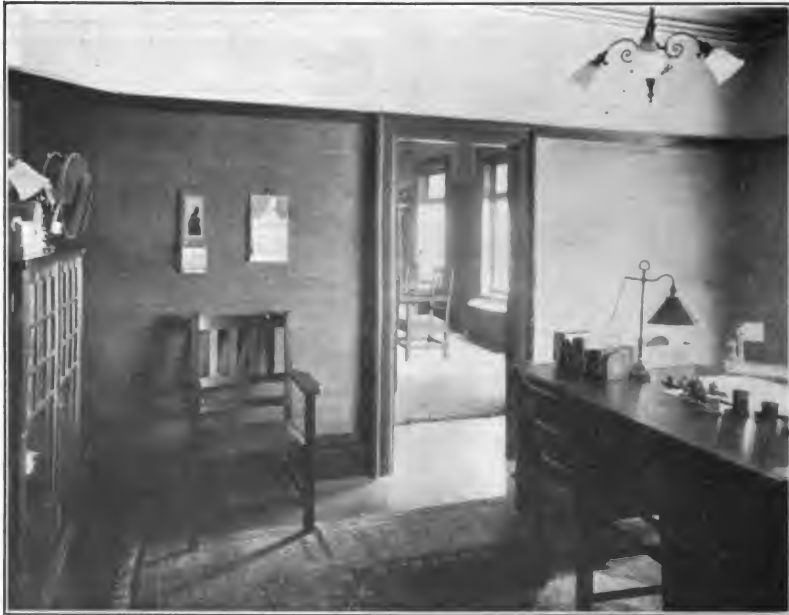
General Manager's Office and Board Room. The Crown Bank of Canada, Toronto.
